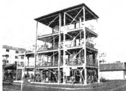
Fig.1 Pilot plant (MITSUBISHI HEAVY INDUSTRIES, LTD.)
